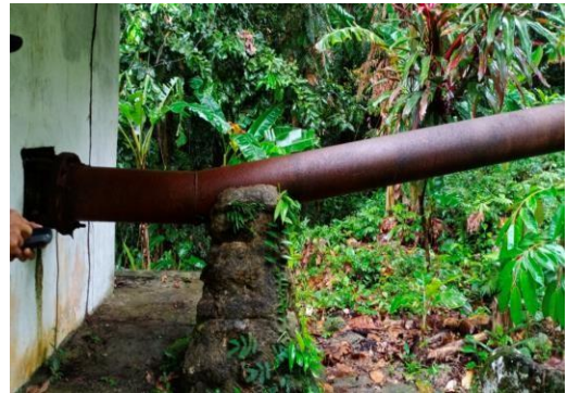
Gambar 7. Pipa Pesat ( Penstock )
