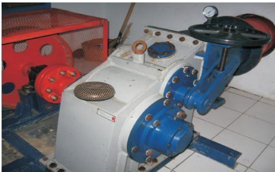
Gambar 9. Turbin Crossflow
