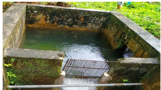
Gambar 4. Bak Pengendap ( Sand Trap )
